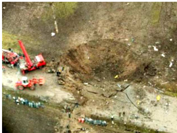
Fig. 3. View of the crater following the AN truck explosion in Romania (2004).
