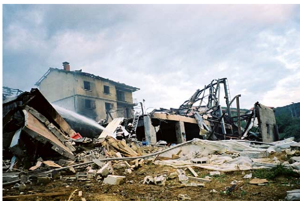
Fig. 2. Ruins after the accident at Saint-Romain-en-Jarez (2003), France.
