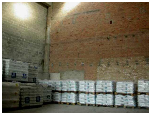
Fig. 1. View of a dedicated facility for AN-based fertilizer storage.
